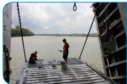
Cadets spent two days cleaning, scraping, and painting, including the most historic feature of the ship, the loading ramp.
